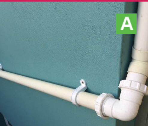
Pipework in Good Condition: Grade A
