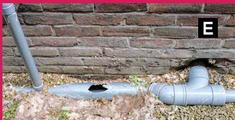
Damaged Pipe: Grade E
