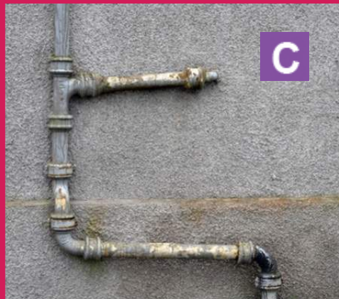
Old and Worn Pipework with Clear Erosion: Grade C
